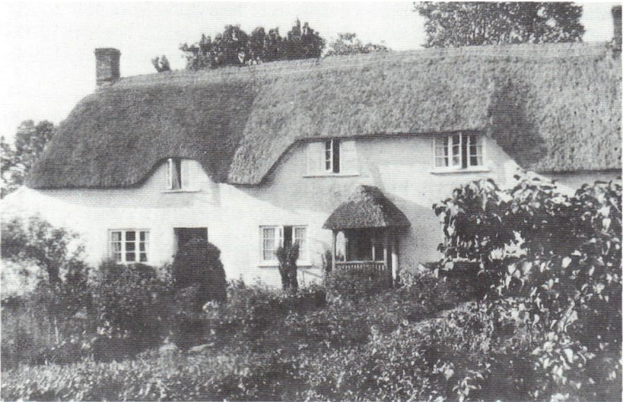
The Cottage early 20th century when it was two dwellings with a thatched roof
